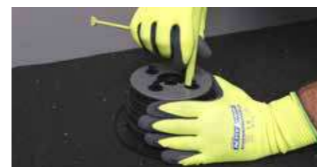
4. Remove pedestal tabs where necessary to accommodate grid positioning along the perimeter.
