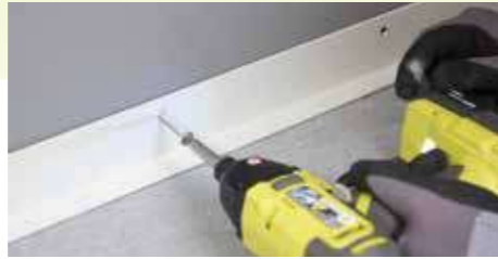
16. Secure the profile to the wall using fasteners.
