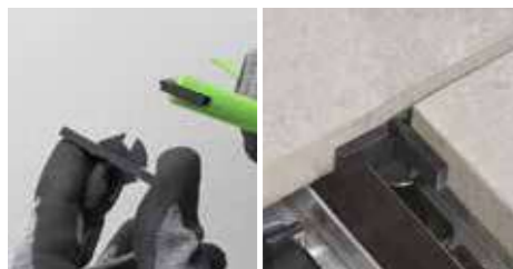
16. Insert the SUPDGS spacers (removing unnecessary tabs) into the slot on the joist where the staggered tile of the next row will be installed.
