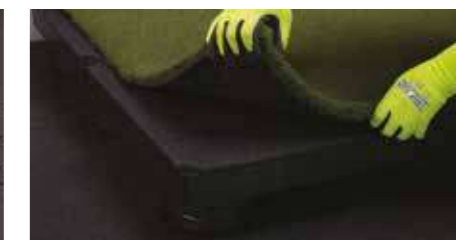
9. Lay the artificial turf roll over the assembled grids, ensuring full coverage and correct orientation.
