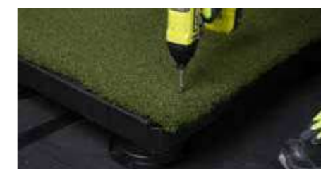
10b. Alternatively, fasten the artificial turf using stainless steel self-tapping screws. Drive screws into the perimeter frame of each grid, every 15 - 20 cm (6 - 8"). Pre-drill if required to avoid frame cracking.
