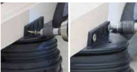
13. Screw the wood joist to the pedestal through the specific slots (use a screwdriver).
