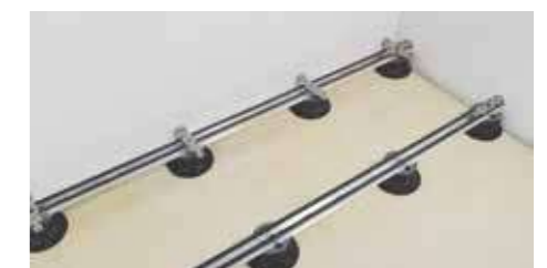
9. Complete the installation in the whole area.
