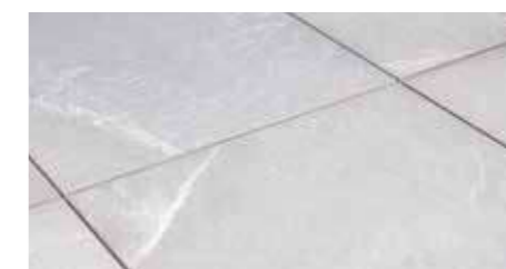
14. Raised floor completed.
