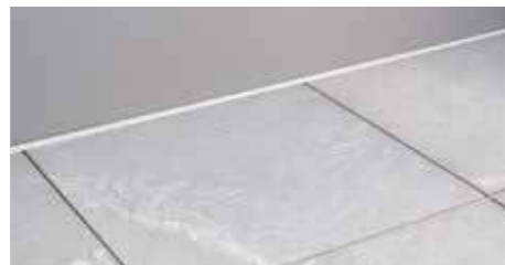
19. Raised floor completed.
