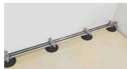
7. Place the remaining pedestals.
